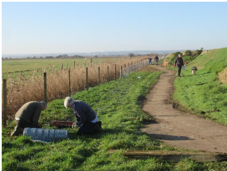
Fencing the entrance path February 2020
