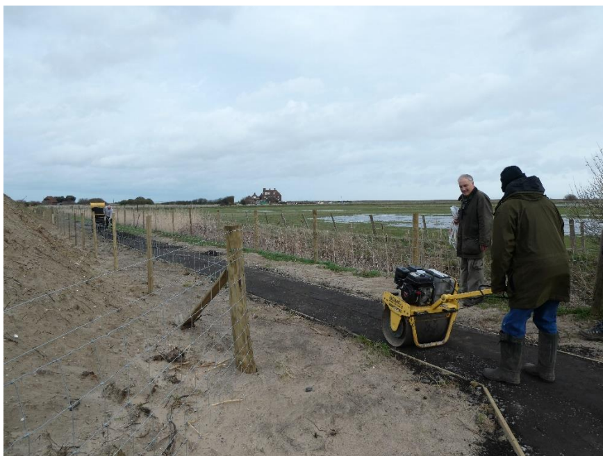
Helping with the laying of the new path
