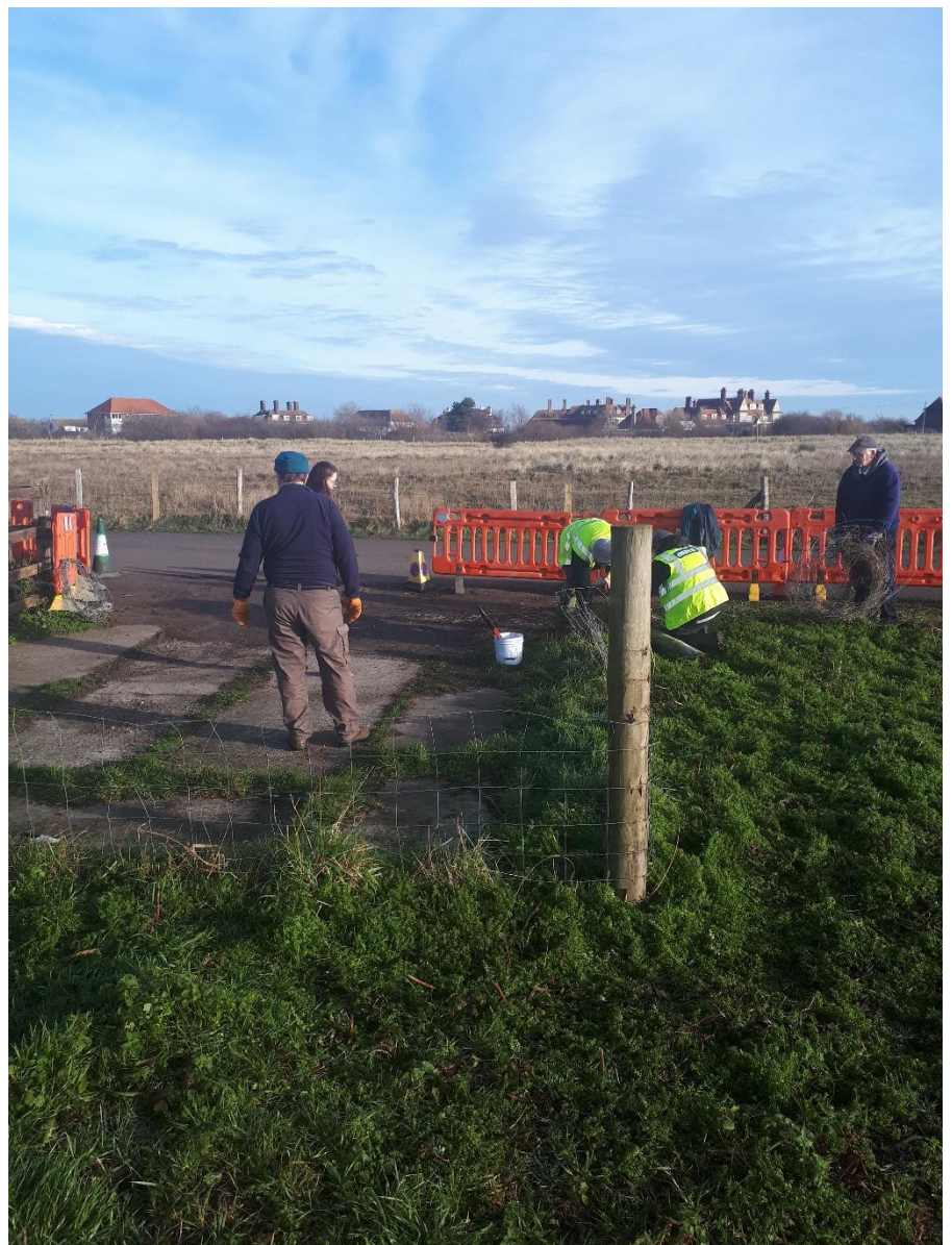
The conservation team removing old fencing and clearing the ground for the new car park area January 2020
