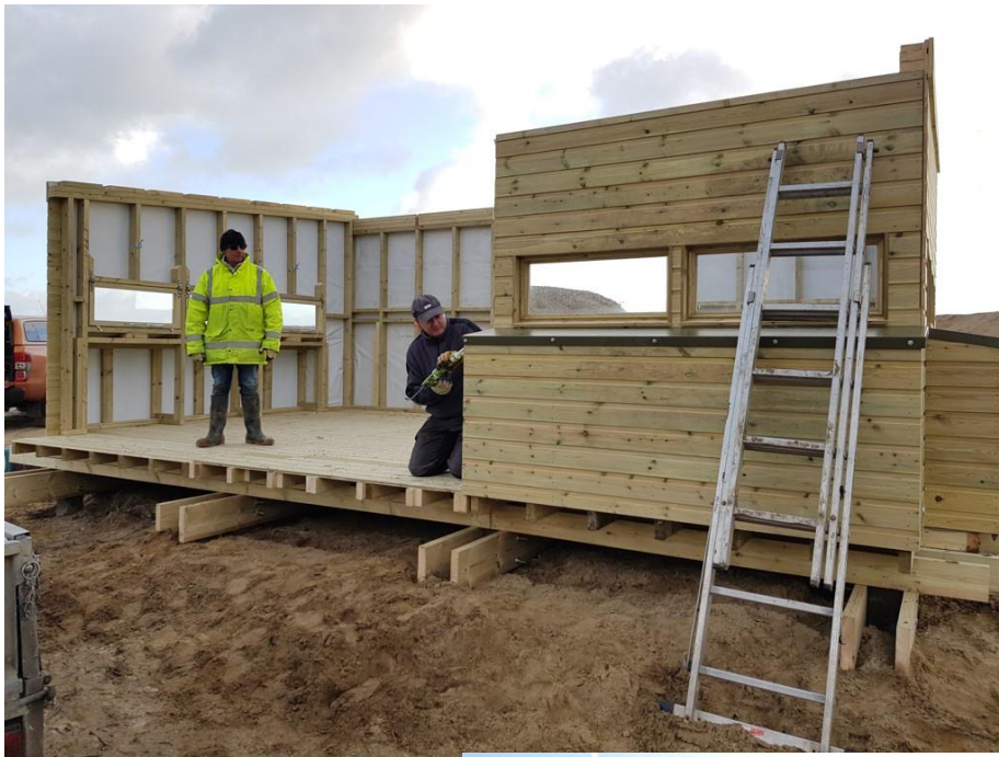
Erecting the bespoke hide October 2019
