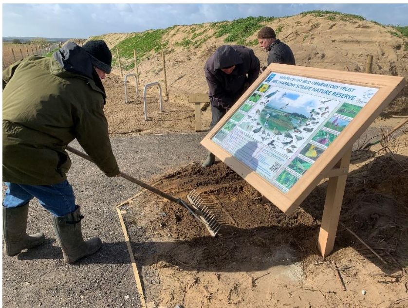
The path complete and bike racks and information board in place March 2020
