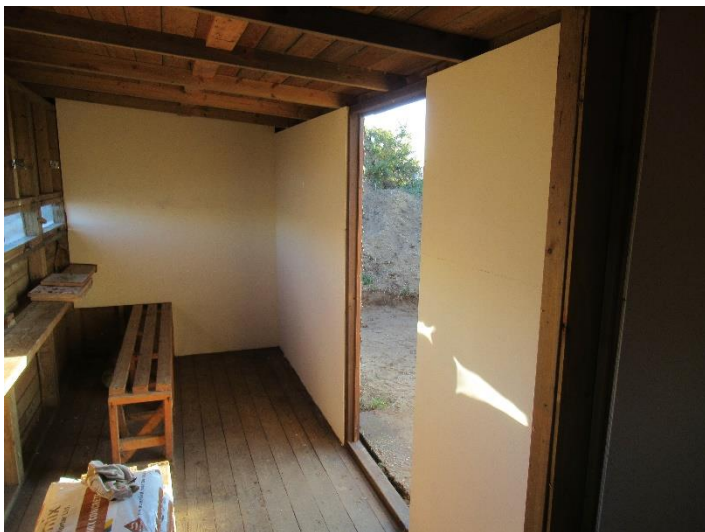
And after internal refurbishment February 2020
