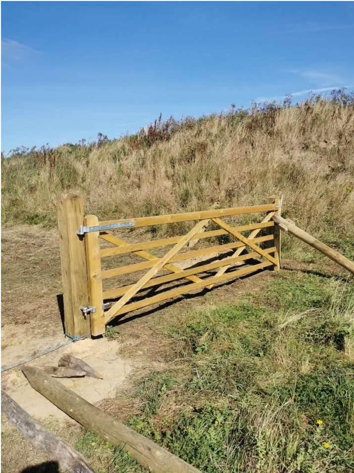
The gate to the meadow area being erected September 2021
