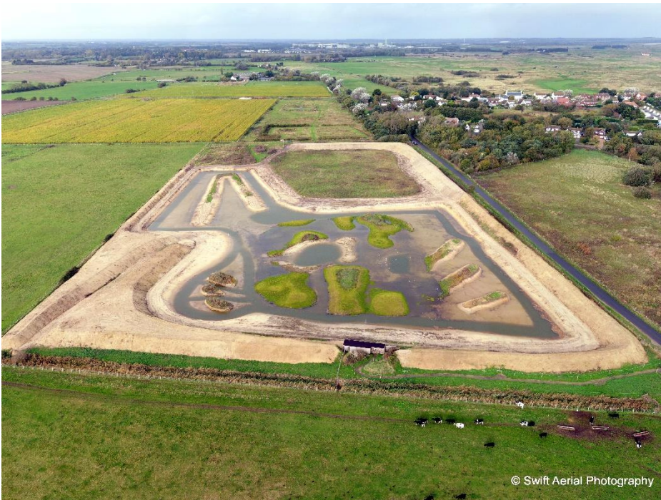
September 2019 Immediately after re-sculpting and before rain filled the enlarged area
