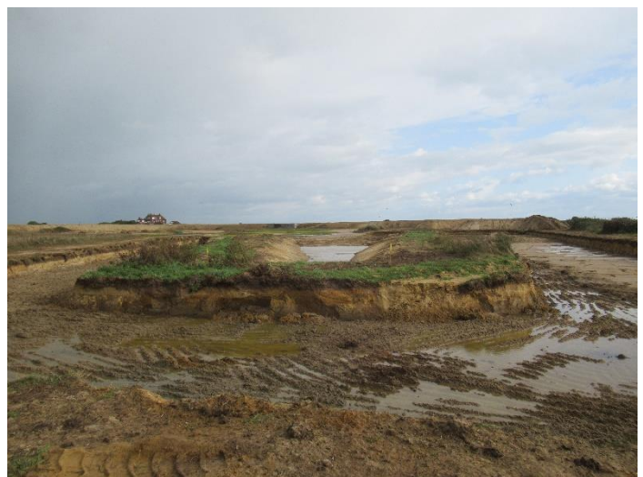
The V shaped island almost complete
