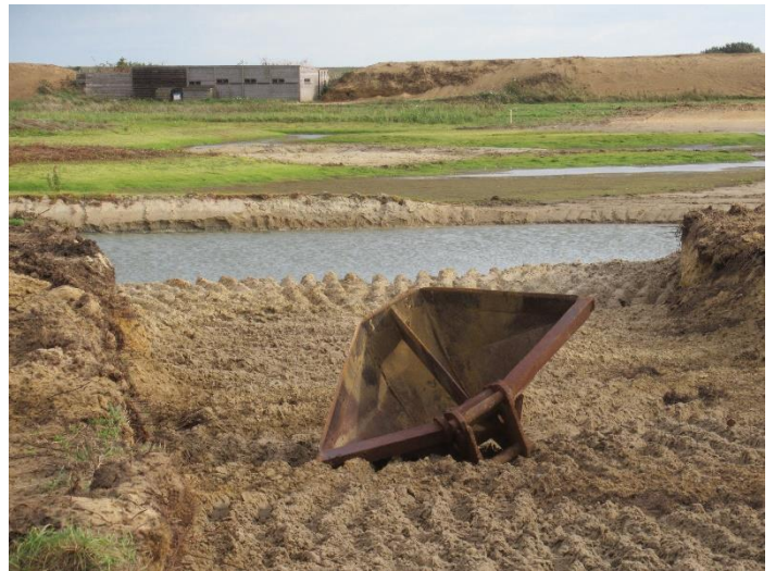
The special tool for digging the deep perimeter
