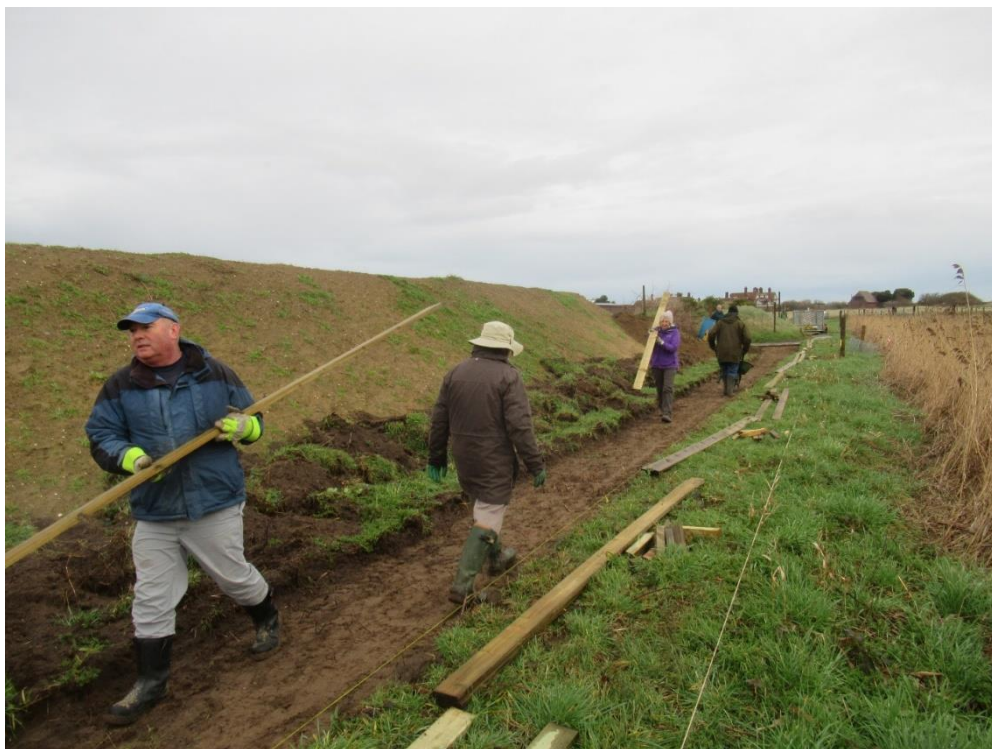
Preparing the shuttering for the new path January 2020
